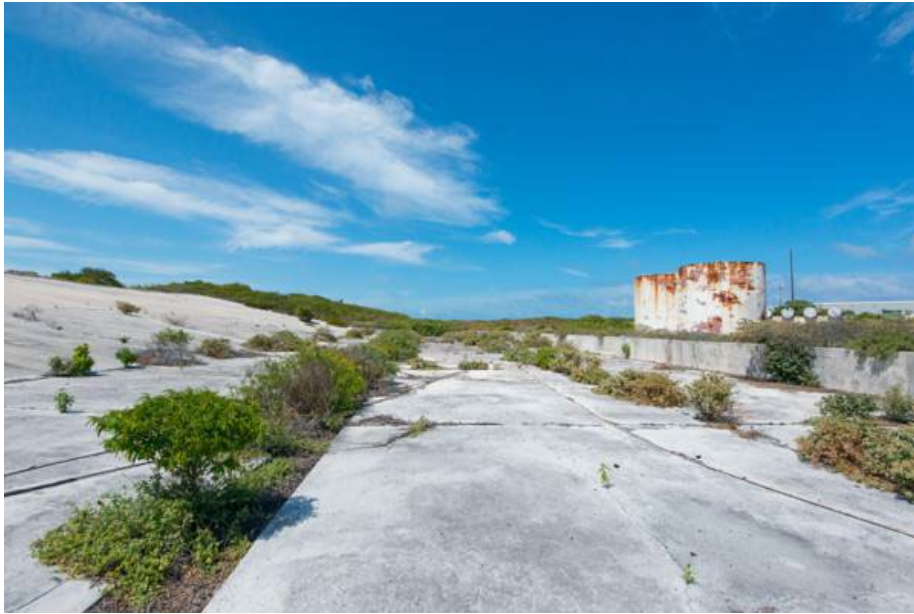
The water catchment area at the abandoned United States Coast Guard LORAN Station, South Caicos.
